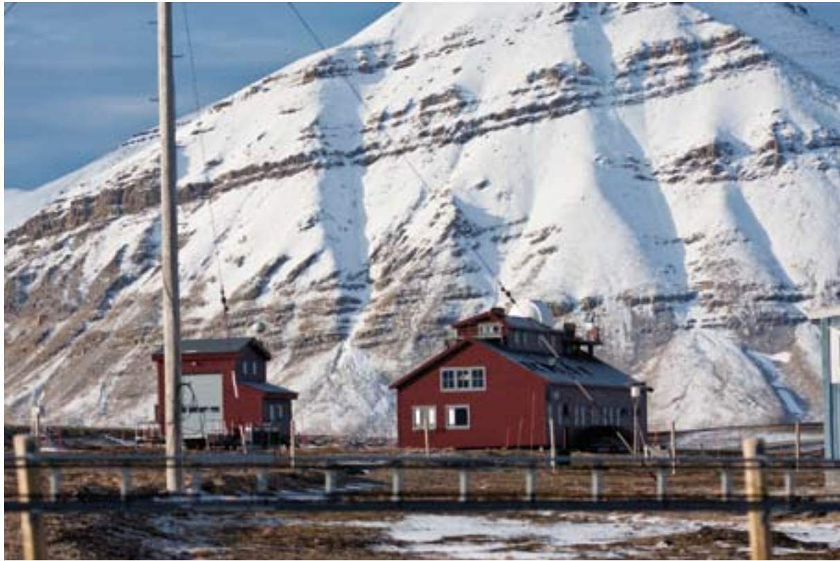
064 | THE ATMOSPHERIC OBSERVATORY LABORATORY AT THE SOUTH WESTERN LIMIT OF THE VILLAGE - THE SMALL BUILDING IS USED FOR LAUNCHING WEATHER BALLOONS AND OZONE SONDES
